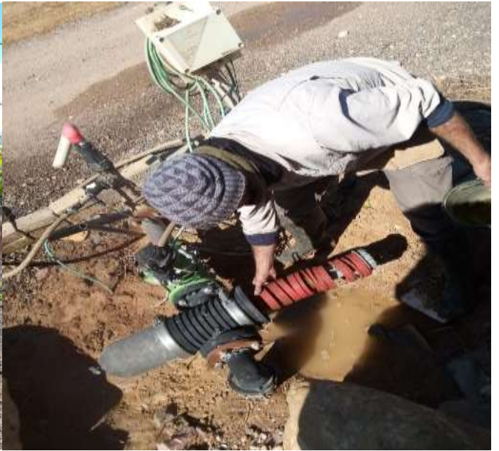
Cleaning of Drip Irrigation Filters
