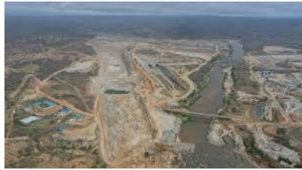
Thwake Dam Under Construction
