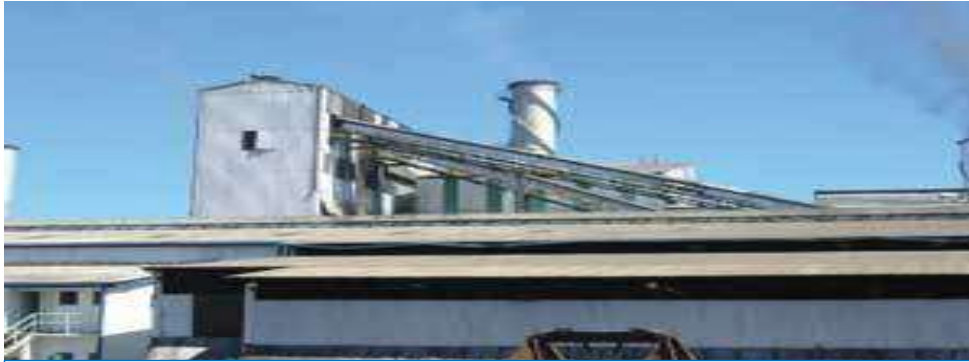
Mumias Sugar Company, Co-generation power plant
