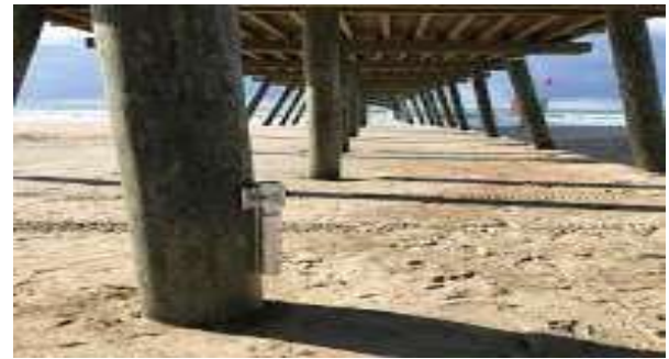
Figure 9.4: Storm-tide sensor installed on a bridge Source: USGS
