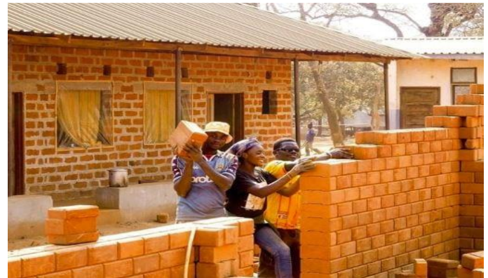
Figure 7.6: Construction of houses using soil stabilized blocks in rural areas Source: Engineering for Change
